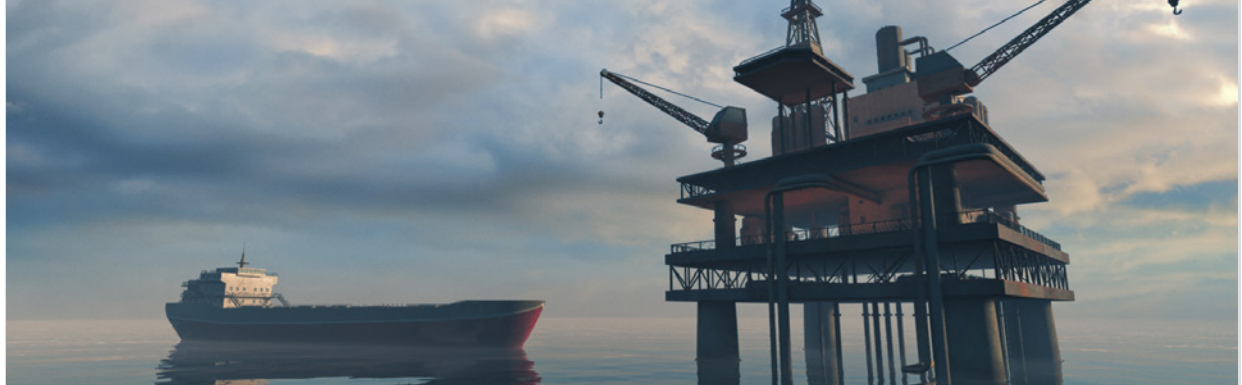
Praxair coatings help protect vital parts of the largest oil development in the Republic of the Congo
